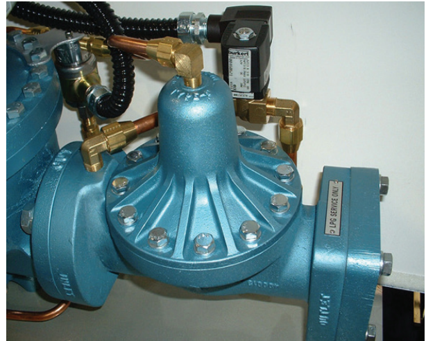
Figure 3-5. Dual Stage LPG Valve
