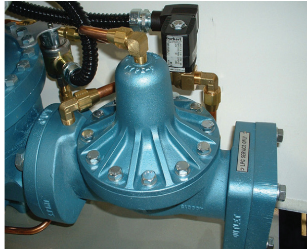
Figure 3-6. Dual Stage LPG Valve
