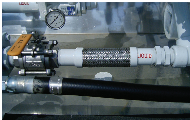
Figure 4-3. Flexible Hose at Outlet
